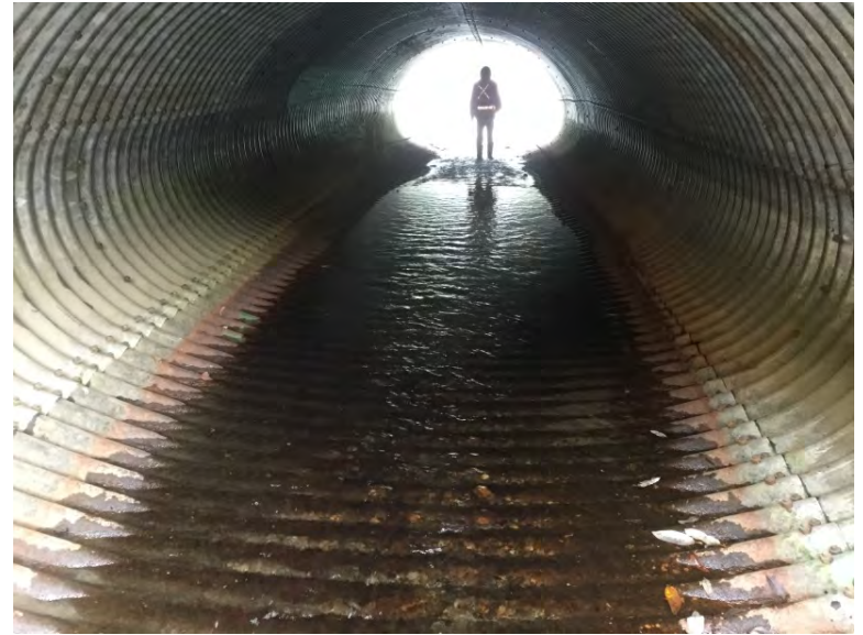
Looking through culvert from inlet
