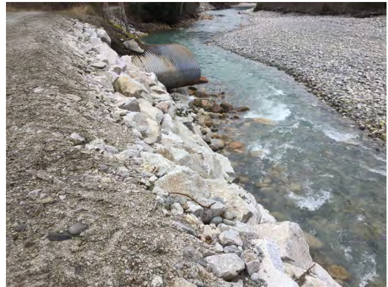
Downstream right approach fillslope
